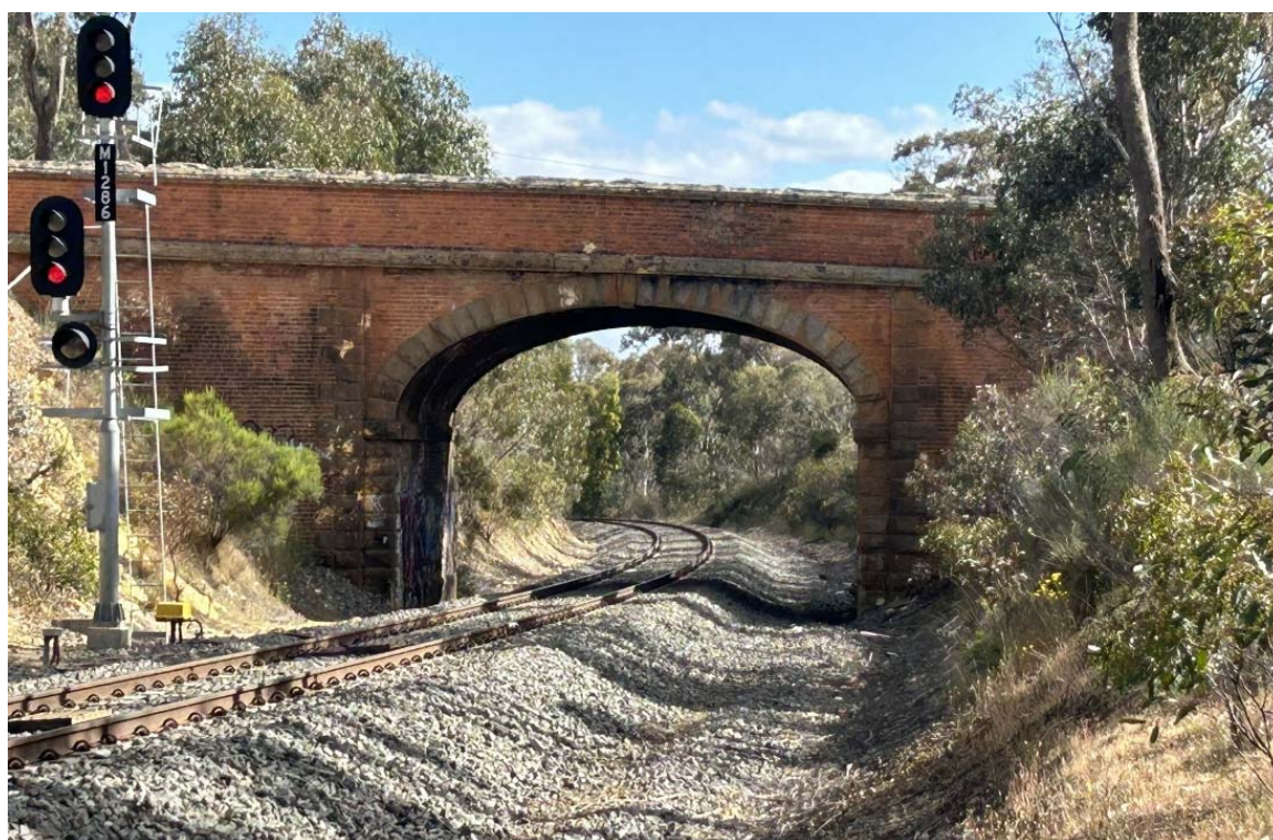
Sawmill Road Bridge over the railway line — Photograph by Andrew Hutchison
